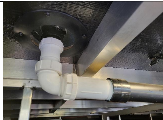
Figure 141. Waterless p-trap under a shower location.
