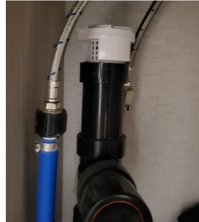
Figure 142. Air admittance valve.
