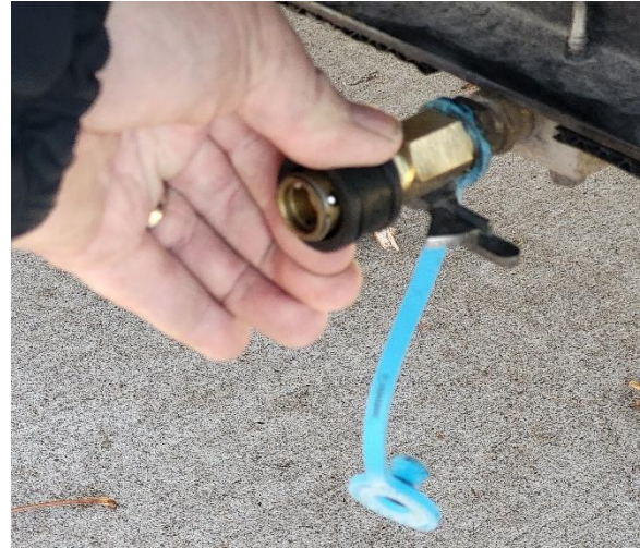
Figure 36. Pushing the retaining ring to accept an appliance connector.
