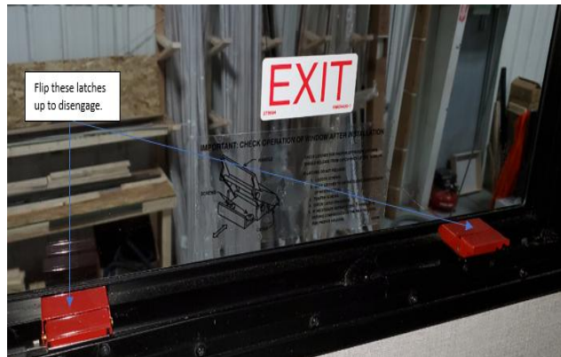
Figure 26. Flip style latch on an emergency exit.
