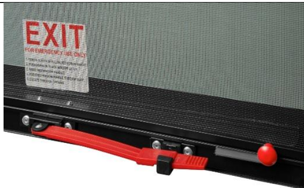
Figure 29. Bar style latch on an emergency exit.
