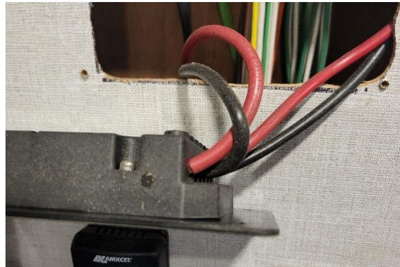
Figure 96. Go Power! Solar Charge controller wiring interface (looking from the top of the controller.). The controller has been removed from the wall and rolled forward.
