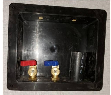
Figure 151. Washer connections and drain.
