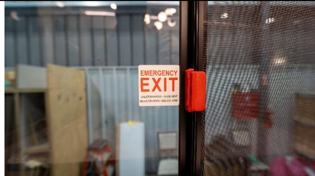
Figure 24. Pull style latch on an emergency exit.
